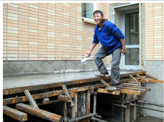
On the Job Training on a Jiguur Construction Site
